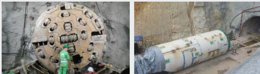
HK Made, Double Shield Hard Rock, Φ 4200 mm, Tunnel Length≈ 3500 meter
